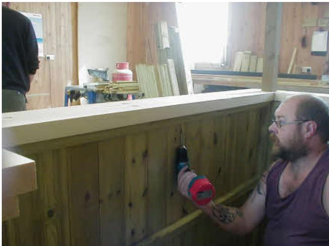
Screw the bar tops into place from underneath the panels as shown. All screw holes are pre drilled.
