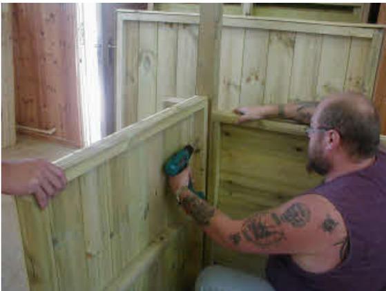
Attach the left hand side panel to the post. All screw holes are pre-drilled.
