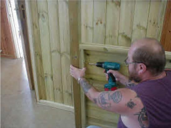
Take the back panel and attach the rear upright post to it. Make sure that the back panel lines up with the inner corner of the post. All panels have to line up with the inner corners of all the posts
