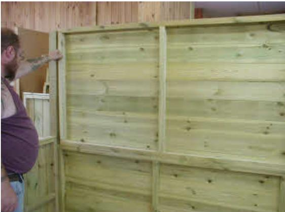
The upper back panel can now be placed on top of the lower panel and screwed to it making sure the the frames are flush with each other. Then screw the upper panel to the rear post.
