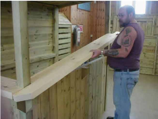
Place the bar top onto the front panel.
