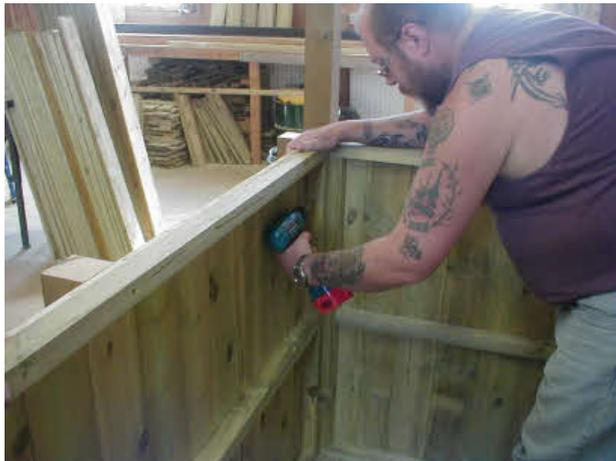
Place the front corner post flush to the side panel and screw into place. The front bar panel can now be screwed to the post
