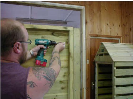
Attach the rear post to the right hand side of the bar and screw into place making sure that the panel is flush with the inner corner of the post.
