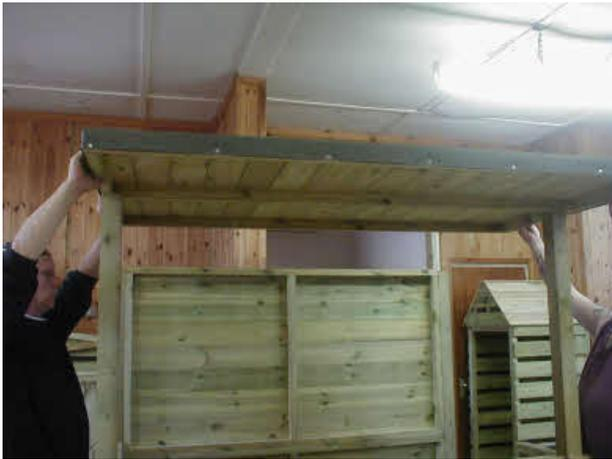
With all four corner posts now screwed into place the roof can be placed on top.
