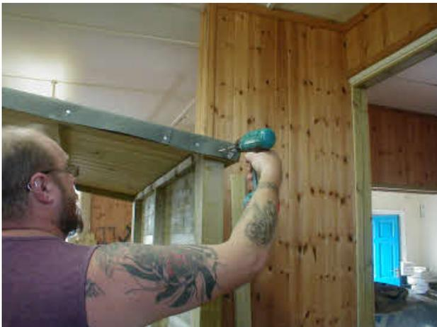
The roof can now be screwed to the rear posts through the **side** of the roof,
